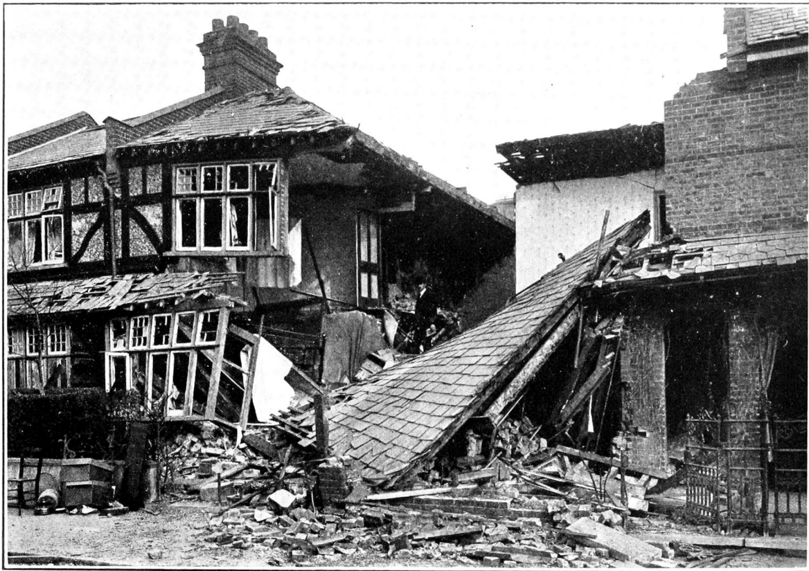
RUINED HOUSES IN EDRIDGE ROAD: Zeppelin Air-raid (13th October, 1915)
